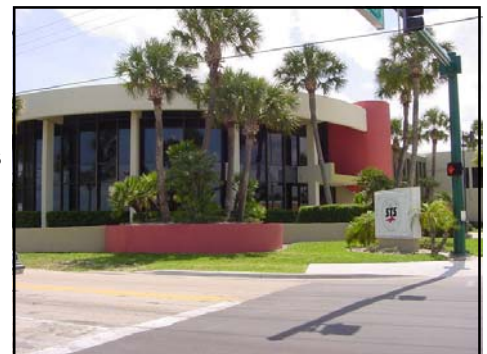
Overlooking the Intercoastal Waterway, the STS headquarters is based in Jensen Beach, FL.
